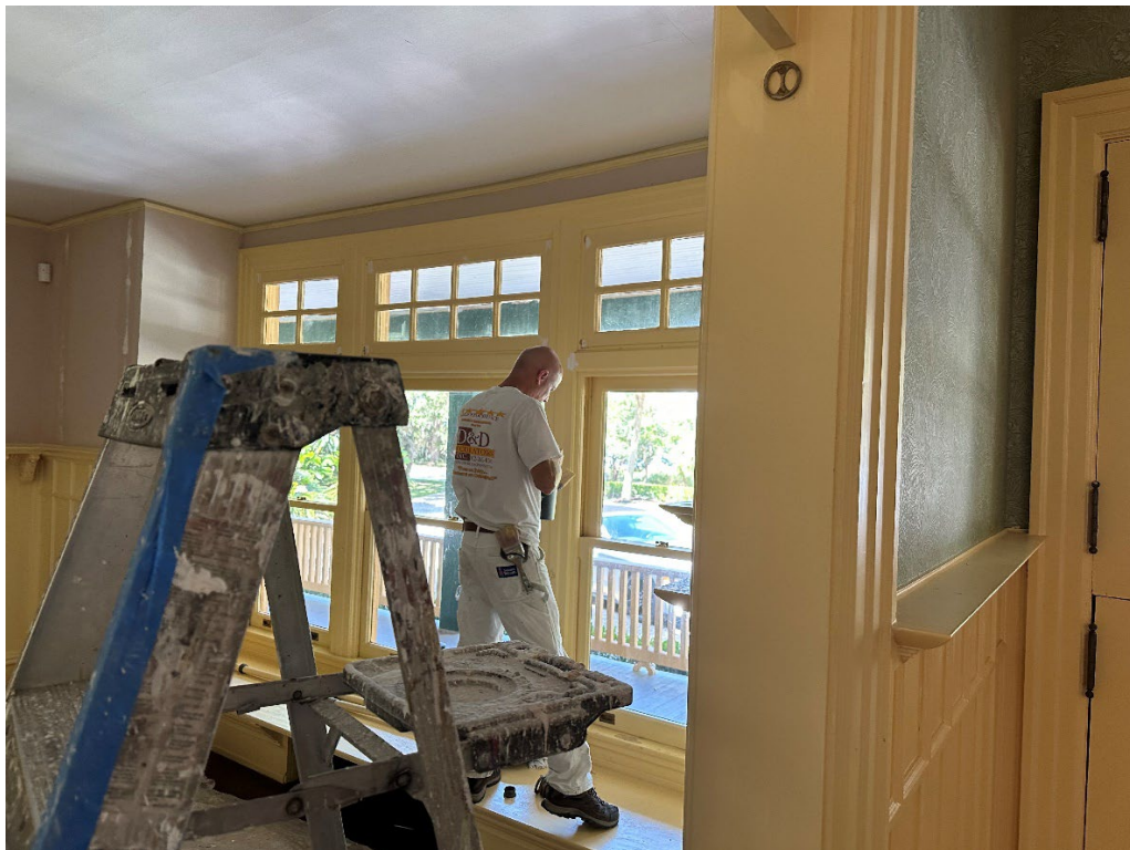
Contractor completing Moss Cottage painting.
