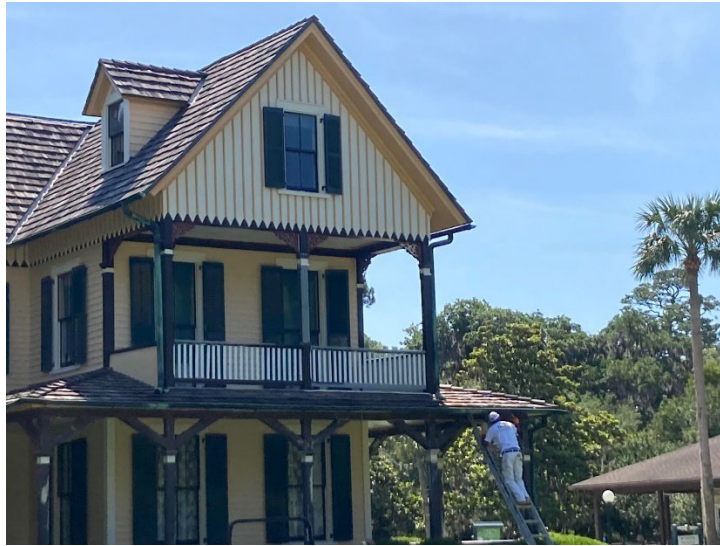
Painting being completed on DuBignon Cottage.
