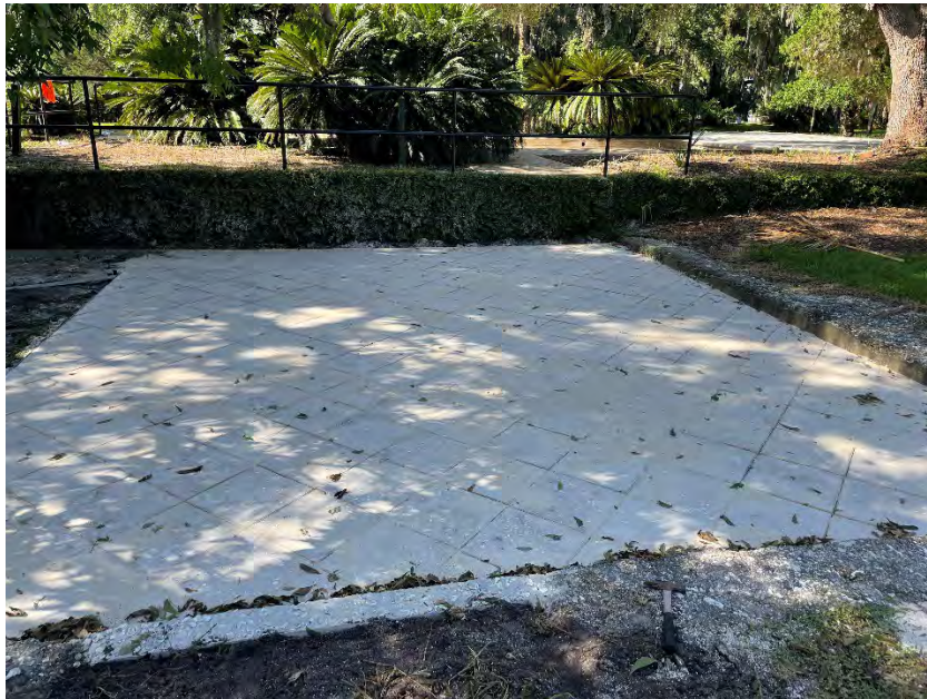
Chichota Ruins work being completed.
