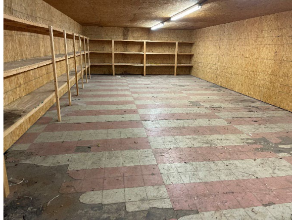
Storage space in Gould Casino prepped for abatement.
